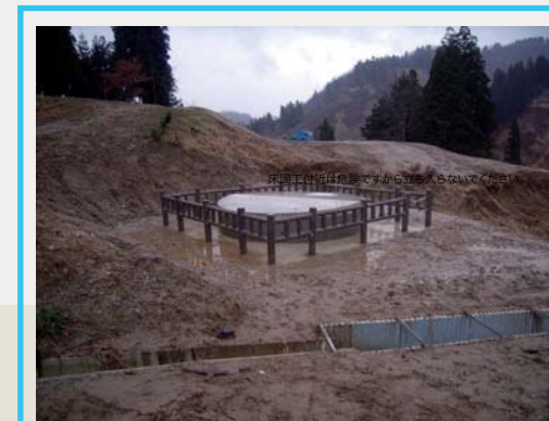
地下水を排水する集水井 Water catchment well (Underground water that causes landslides is collected for drainage.)
