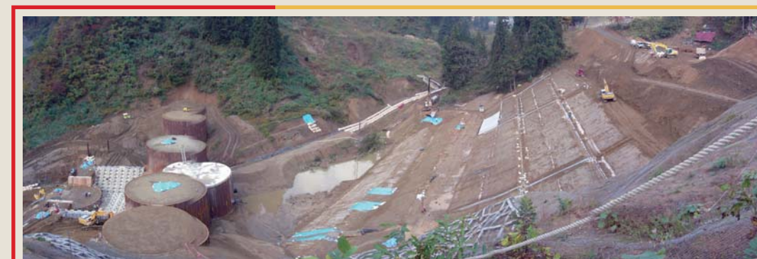
床固工(セル型)と、地すべり土塊を押さえる盛土工。工事の様子。 Groundsill work (steel sell) and filling works to fasten lower part of the landslide.
