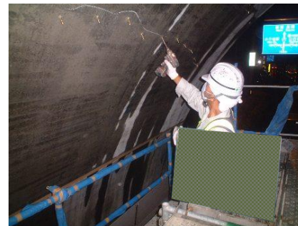
ひび割れ補修（注入）状況
