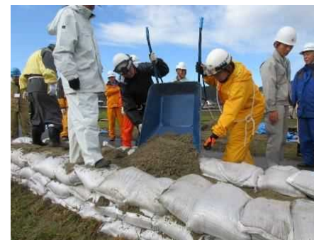
積み土のうエ [水防工法演習等] (図3.4.12)
