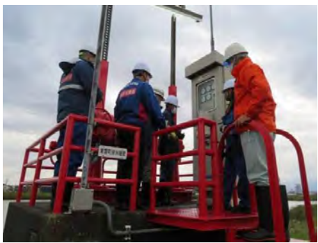
排水樋管の点検
