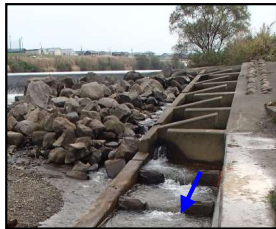
左岸魚道改修前 (H26)
