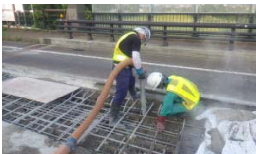
(橋梁修繕：床板打替等)
