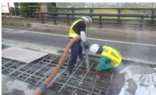
(橋梁修繕：床板打替等)
