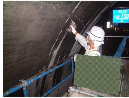
ひび割れ補修（注入）状況
