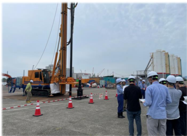
[大規模な工事現場の見学]
