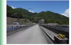
⑤ Omachi Dam levee crown
