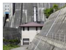
⑫ Omachi Power Plant
