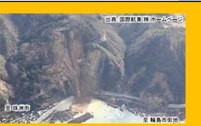
Photo 1: Major landslide in coastal area of NR249
