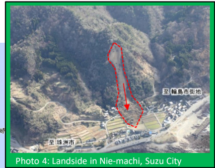
Photo 4: Landslide in Nie-machi, Suzu City
