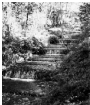
French style stepped dam in the Ushibuse-gawa River (Work executed by Nagano prefecture under the national aid granted after the sabo law was enforced in 1897).
