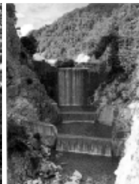
Japan's first arch sabo dam. Sabo dam in the upper reaches of Kamagafuchi
