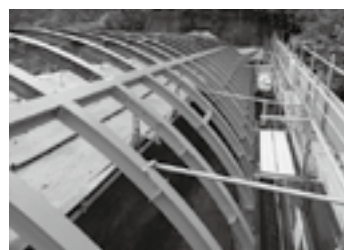
補修工事状況 ▶P.13
