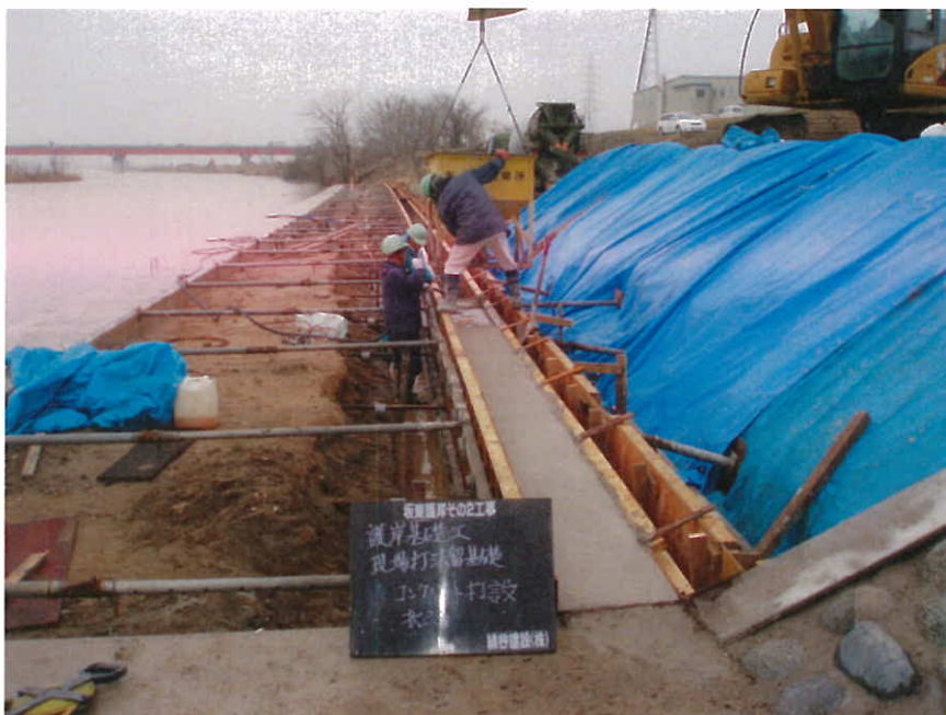
(参考) 庄川：板東護岸工事
