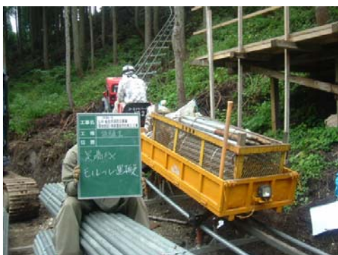
(資材運搬状況)
