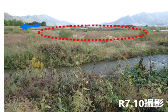
左岸83.0k付近
