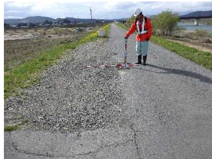
堤防天端損傷状況把握
