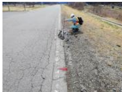
堤防天端損傷状況把握
