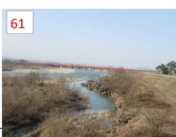
No.86 漏水 漏水 L=5214m 15.8k+100m~20.8k+160m
