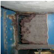
H21損傷状況 (主桁腐食)
