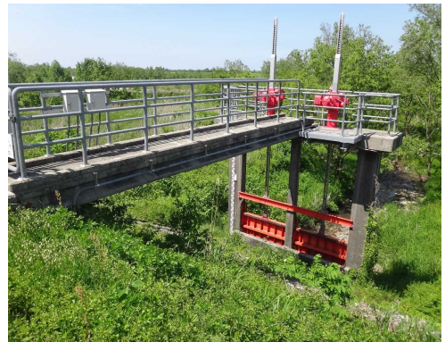
[舟子川排水樋管]
