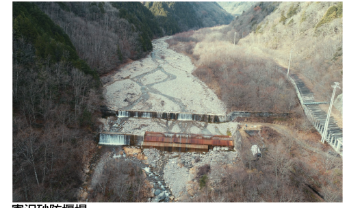
寄沢砂防堰堤
