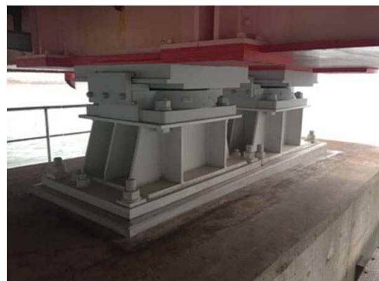
( 補修：支承の更新 )
