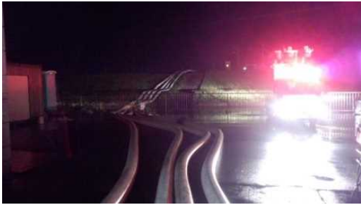
①九竜橋川排水樋管
