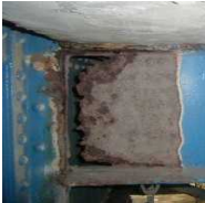
H21損傷状況 (主桁腐食)
