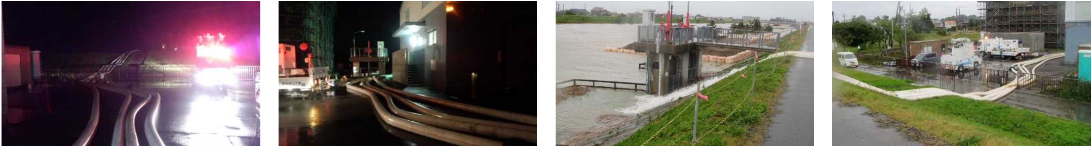
①九竜橋川排水樋管
