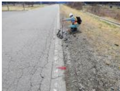
堤防天端損傷状況把握
